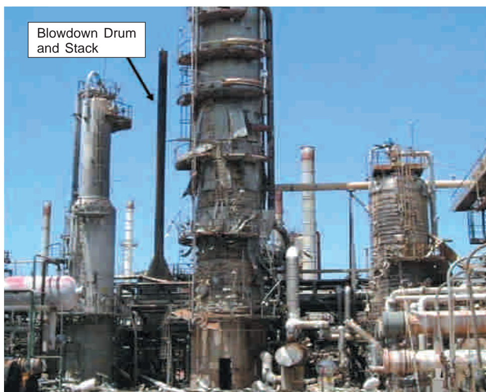
Picture showing the offending blowdown drum and stack that were the initiating points of the fire.
