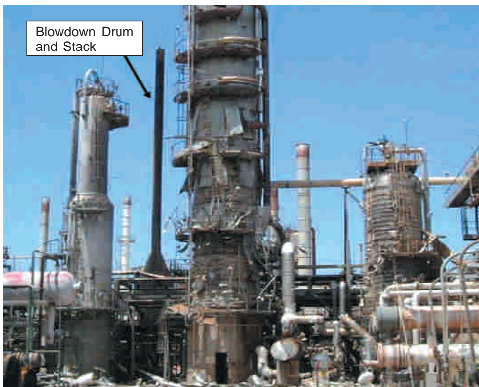
Picture showing the offending blowdown drum and stack that were the initiating points of the fire.
